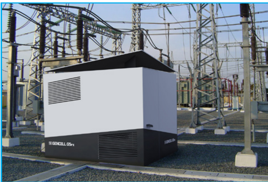
Figures 12: Exterior view of the GenCell G5rx utility backup power solution.
